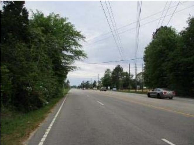
View north along Whiskey Road
